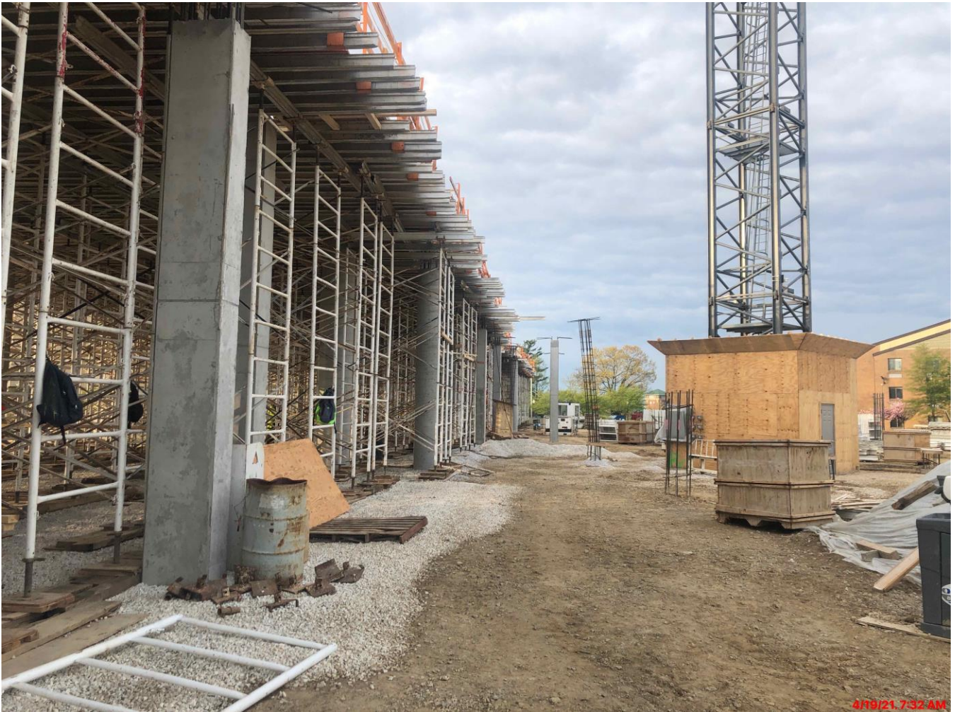
2 nd Floor Construction, Concrete finished, and below framing
