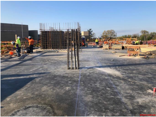
2 nd Floor Construction, Concrete finished, and below framing
