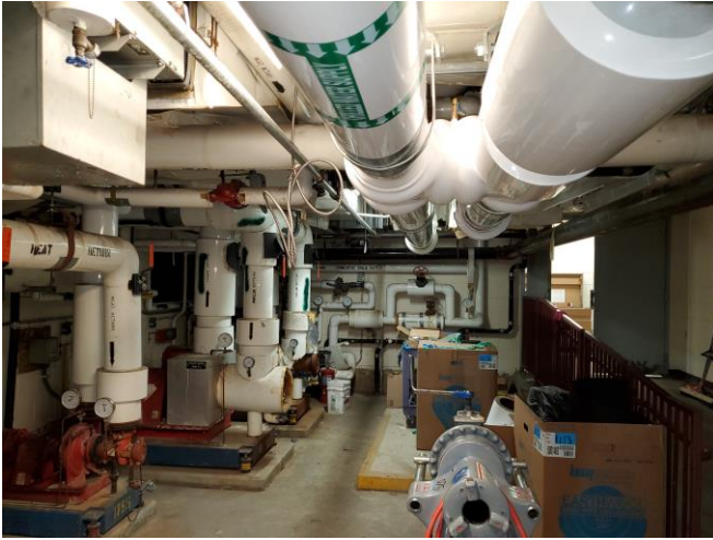
Spencer - Steam Loop McMechen Tie-In:
