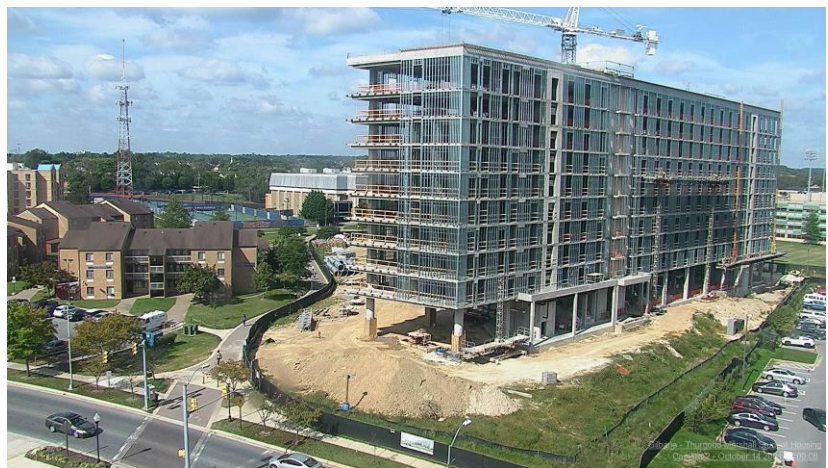
South and East Side of Building with Brick Erection System
