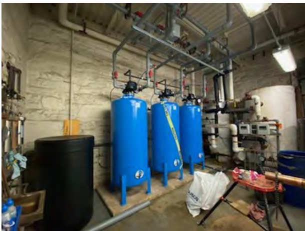
Water Softeners and Typical Electric Meters
