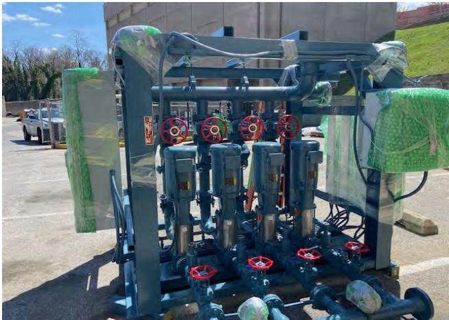
New Boiler Water Pumps – Steam Plant
