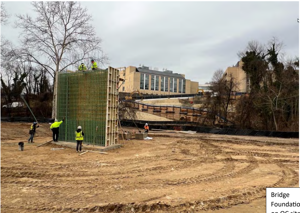
Retaining wall for Bridge. Looking from OC site
