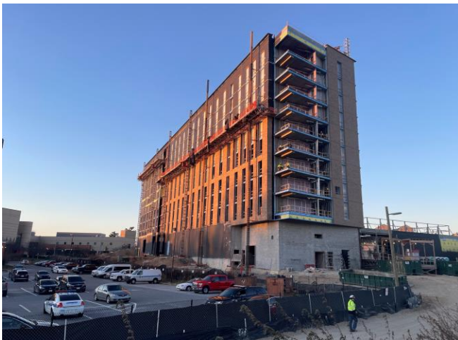
East Side of Building Showing both the North and South Ends. Brick is going up on the east side (north side brick is completed with windows being installed)
