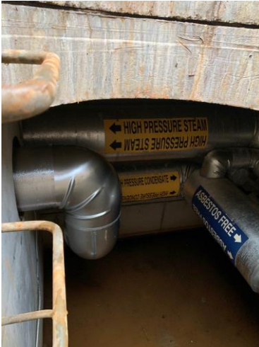
Newly insulated pipes and decayed manholes requiring repair
