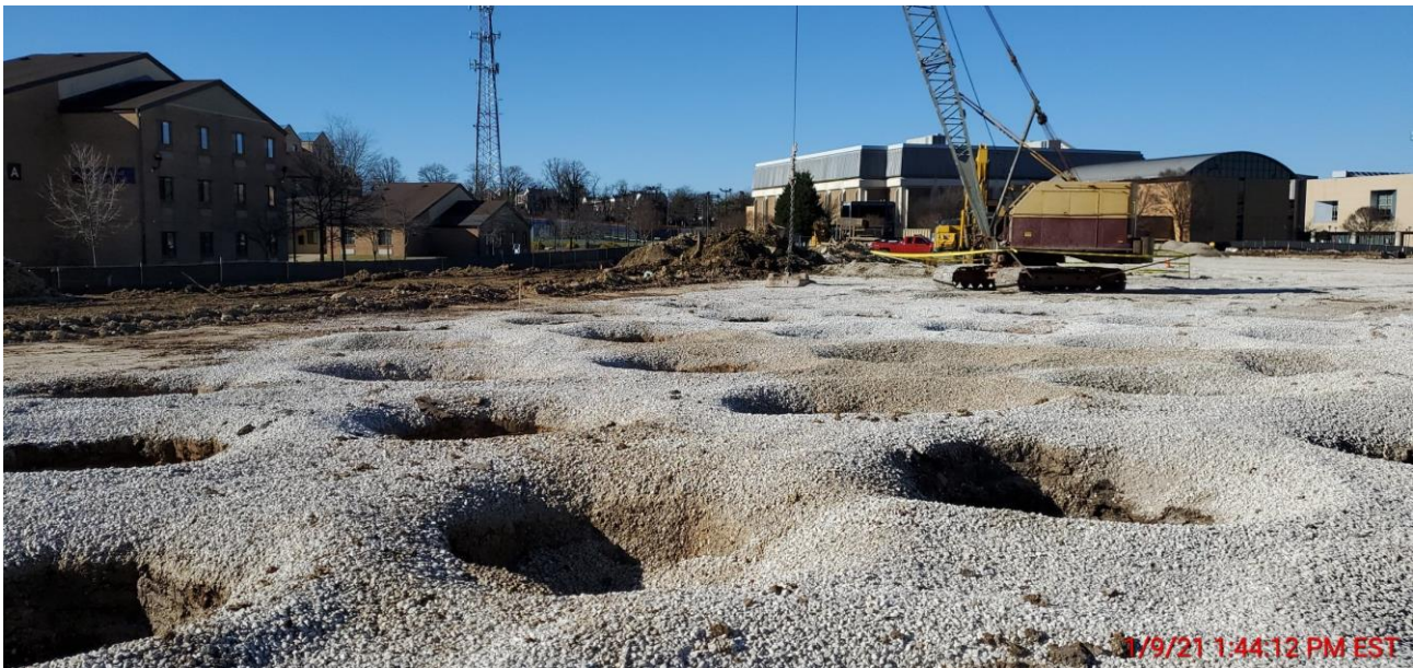
Soil Compaction in Preparation for Caisson Work
