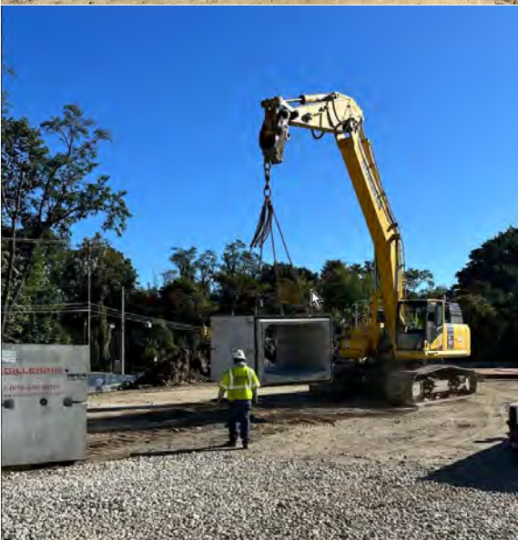
Culvert Sections
