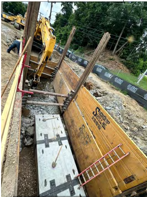
Trench for Culvert
