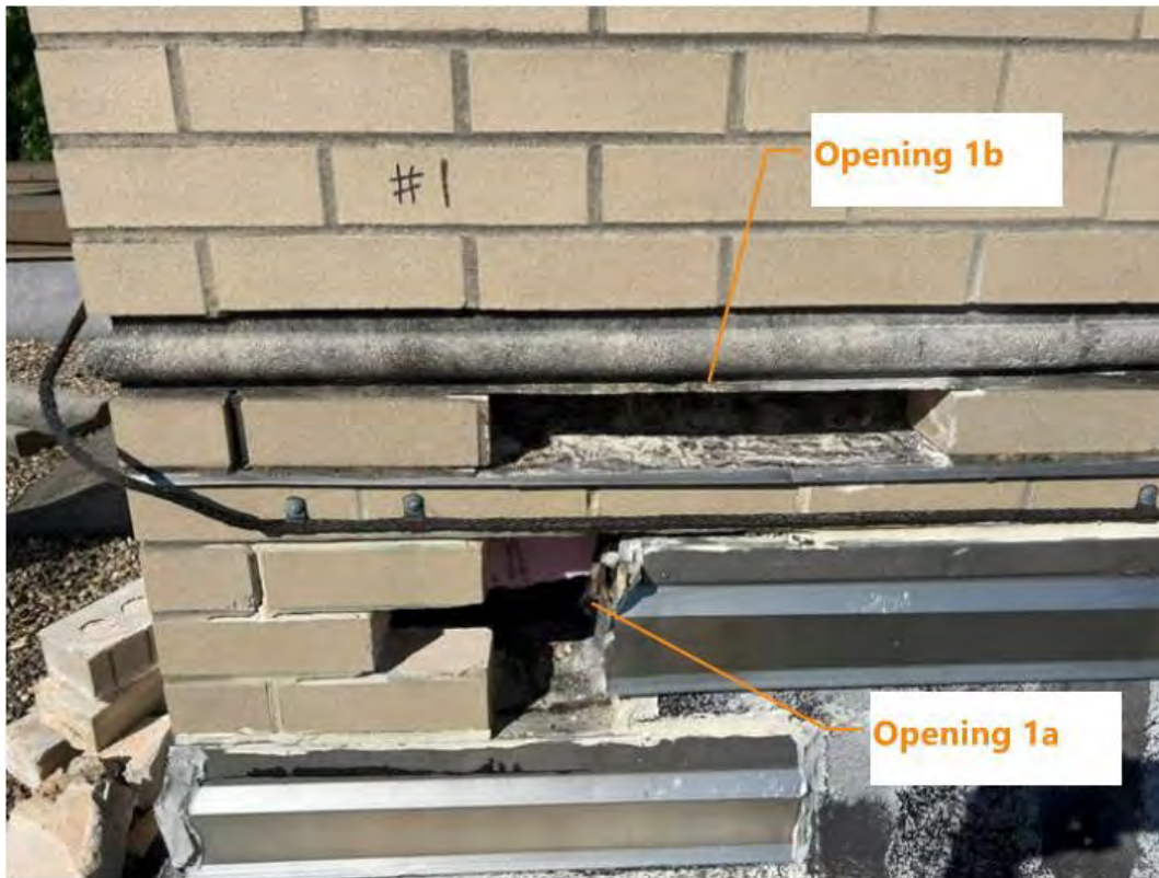
Figure 6. Overall view of Opening No. 1 following limited removal of brick cladding.
