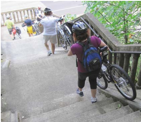
Example of stairway runnel
