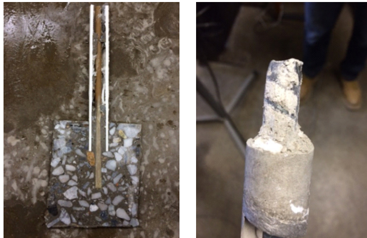
Fig. 12: Inconsistent rebar alignment and bonded length within most specimens
